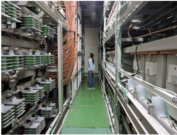
Huge Capacitor Bank System
