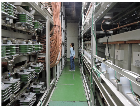
Huge Capacitor Bank System
