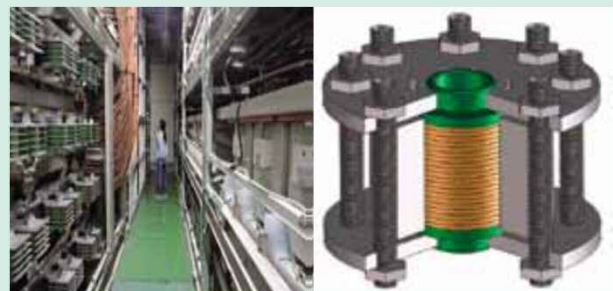
Huge capacitor bank system, and cut-view of a wide-bore pulse magnet
