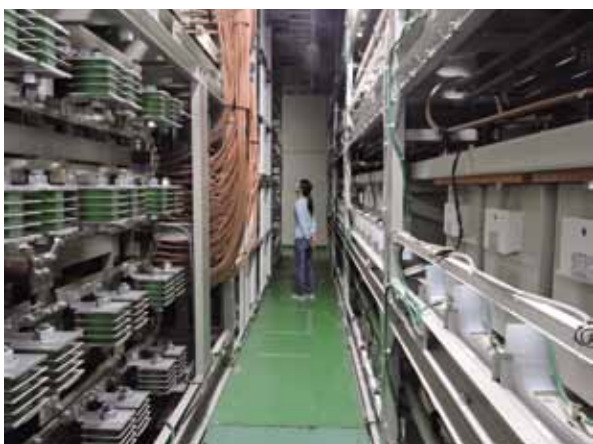
Huge Capacitor Bank System
